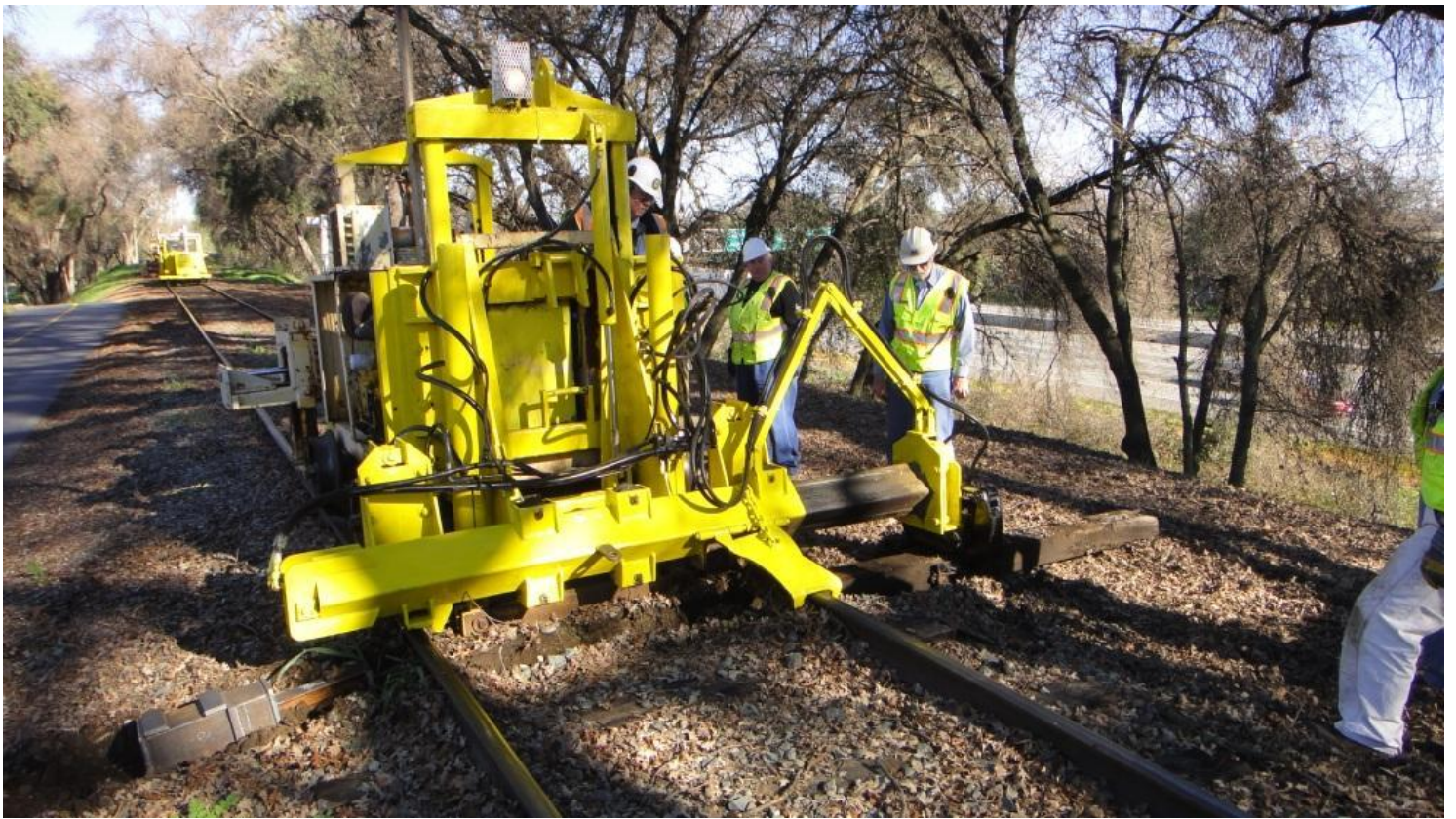
Chris at the controls of the Jackson 125 Tie Exchanger as it pulls its fist tie on the SSRR Main
