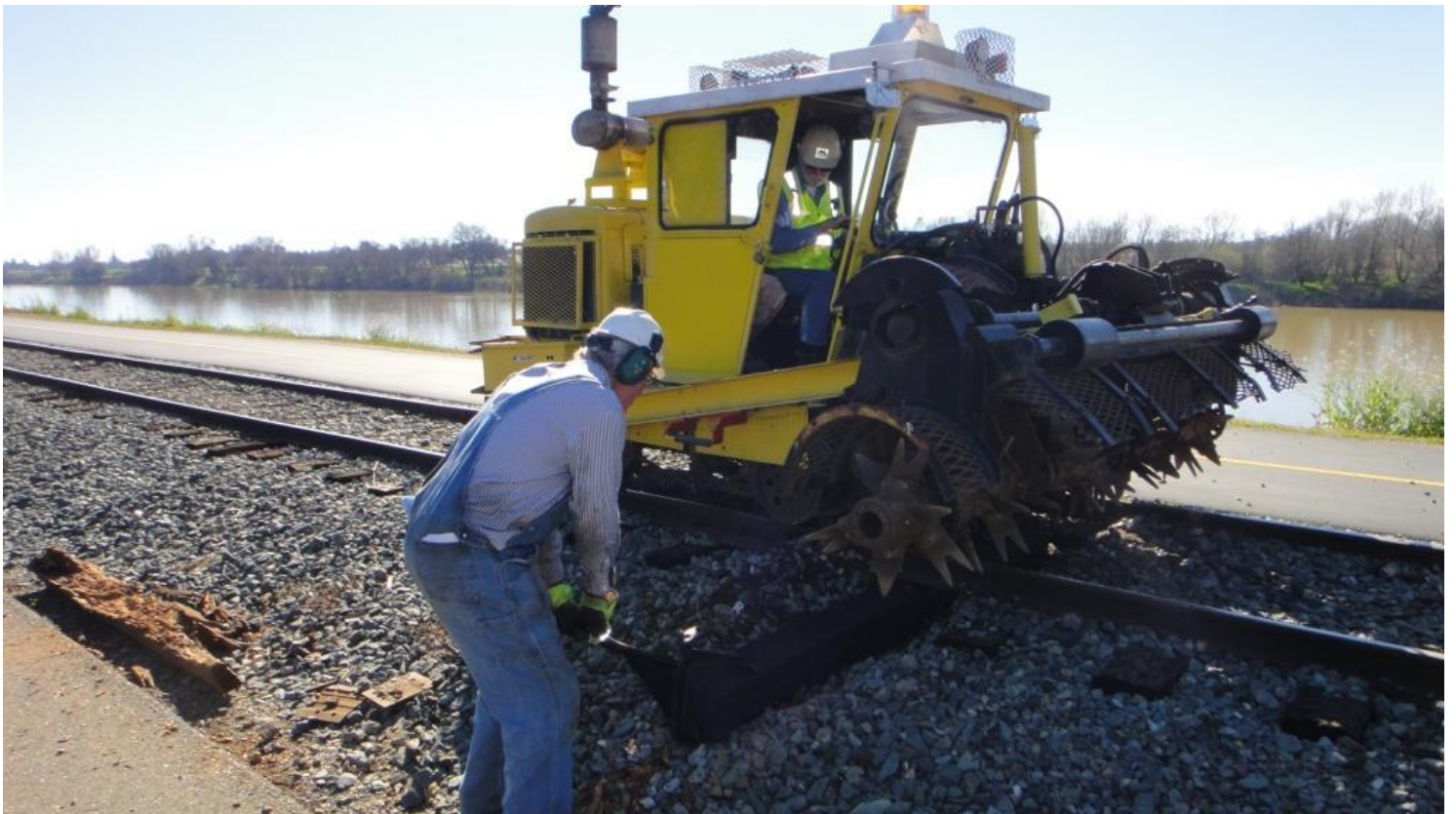
Bring in the scarifier/insertor: Alan at the helm as Steve guides a new tie into place
