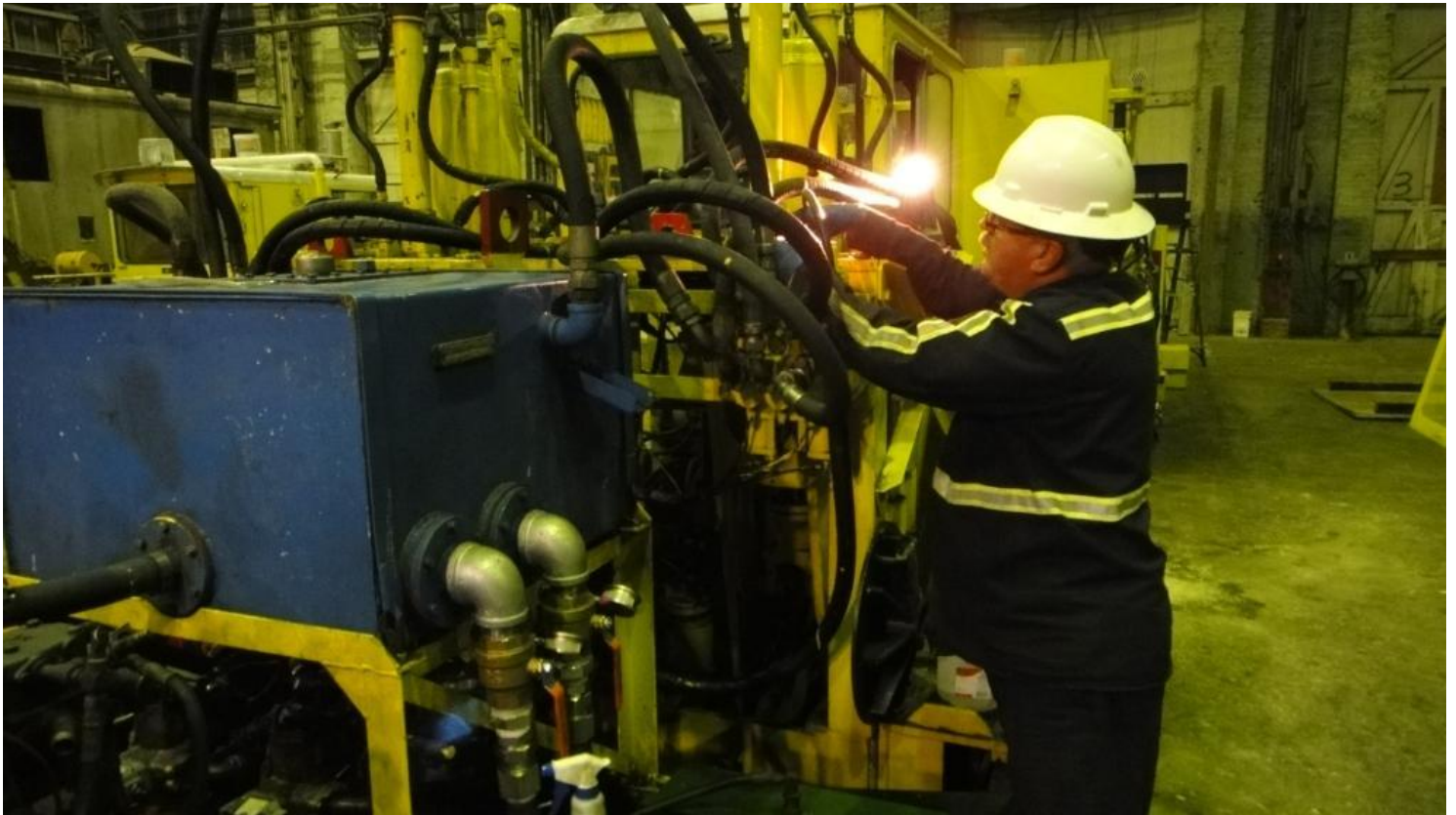
Team Tie Shear's Captain Scott trouble-shoots the compressed air system
