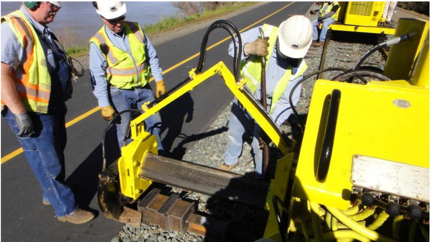
The view from the control cab of the 125 as Chris, Ed, and Mike M. position Cliff's ram attachment to push out tie
