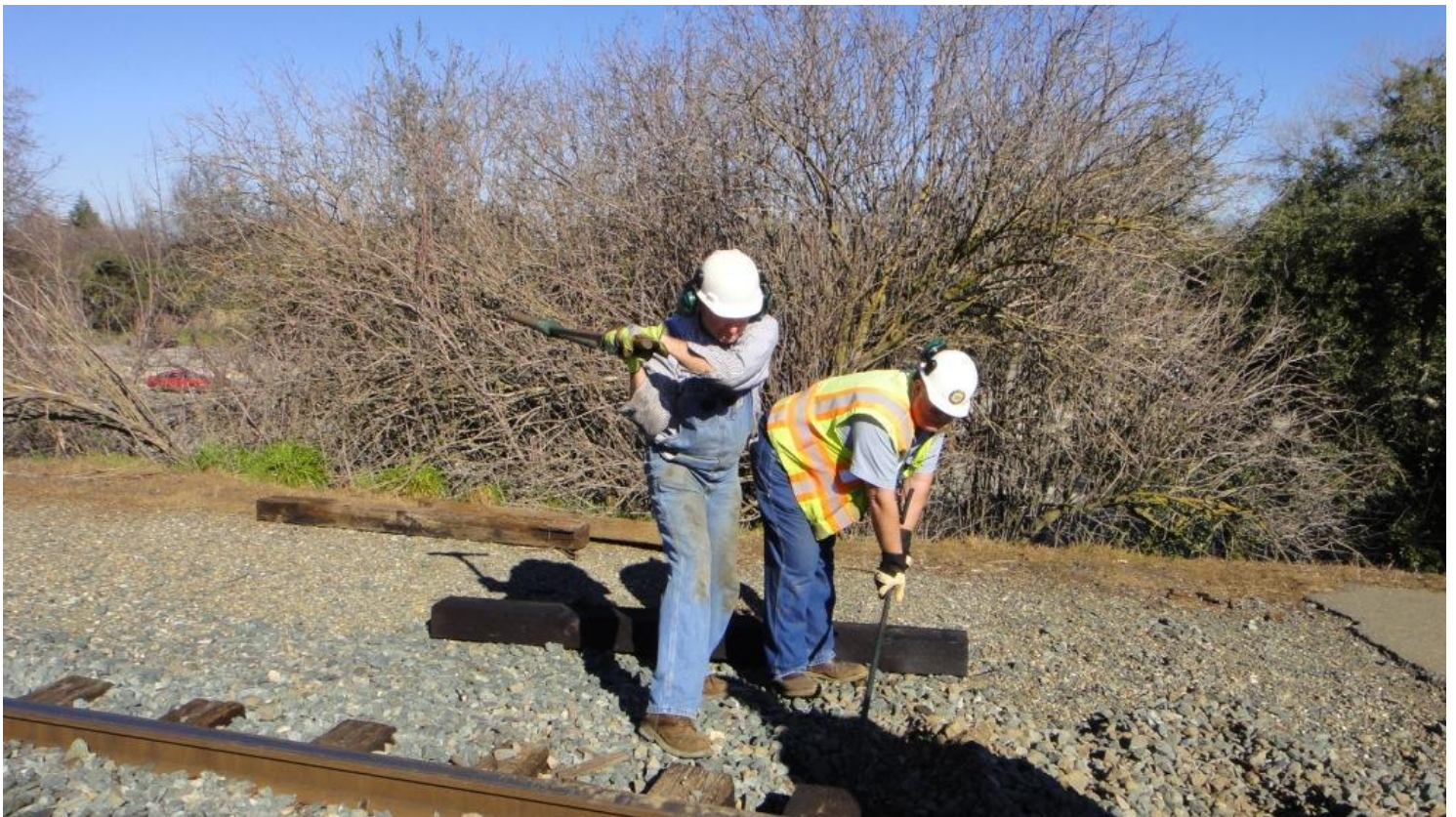
As Chris nips-up the tie, Steve show the proper way to drive a spike with a spike maul
